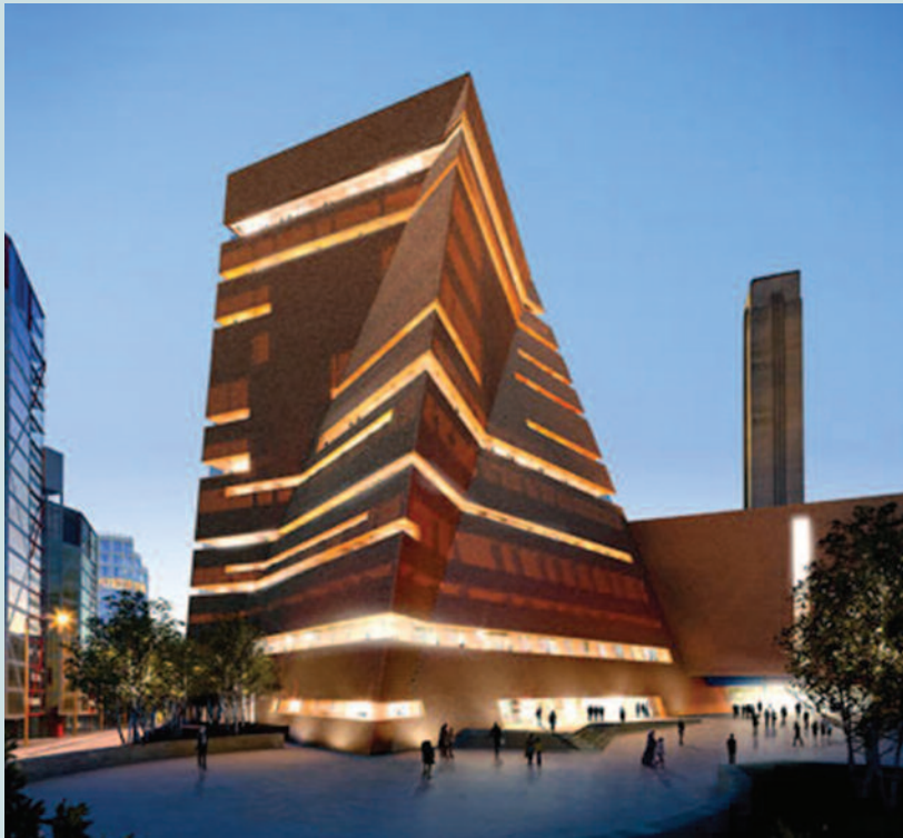
Tate Modern extension, London (currently under construction)
